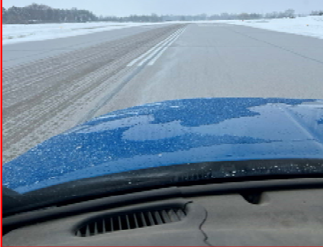
Runway deicing. It takes about 55 gals of deicer to deice the runway 30' wide. This ice-covered runway was down to bare pavement in 1 hour. A few passes with the sweeper and we were back in business.
